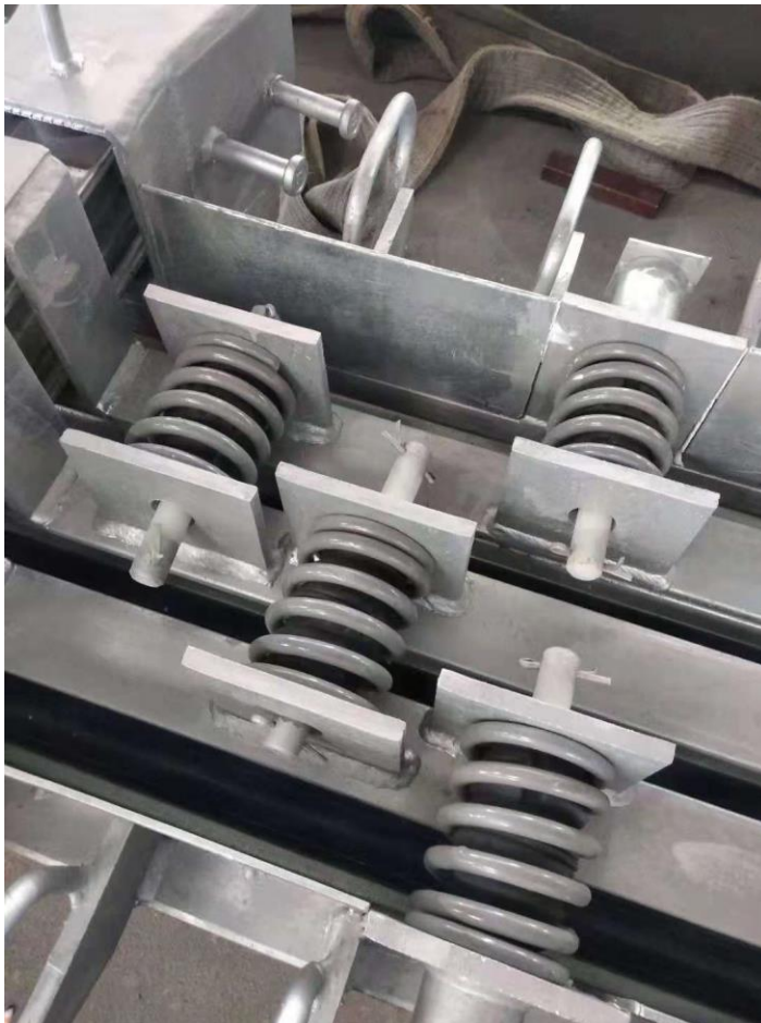
TechStar-Tegu modular bridge joint supporting system
